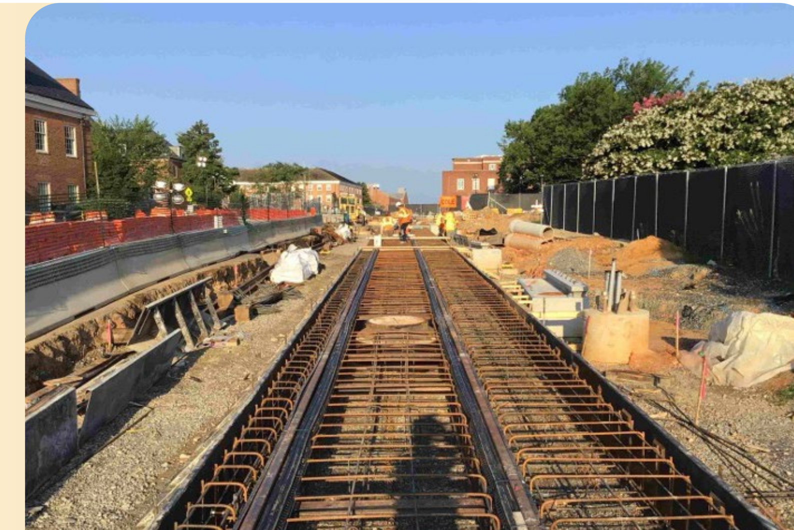
Embedded track construction
