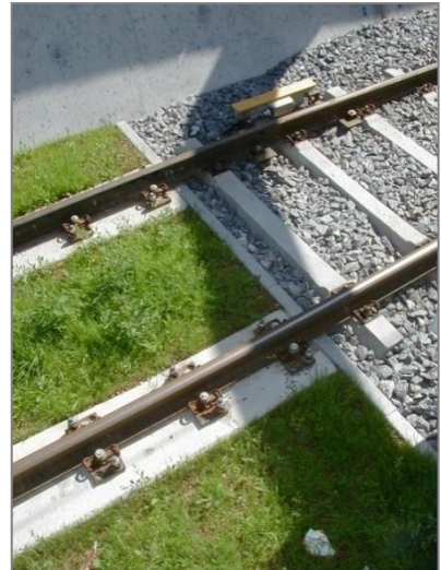
Green track transitioning to ballasted track
