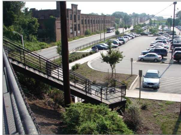
West Baltimore MARC Park-and-Ride Lot, looking east toward Franklin Street
