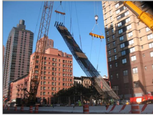
Example of Rebar Cage Installation
