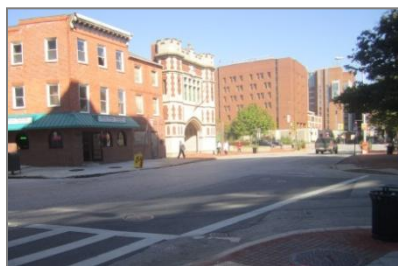
View of Poppleton Fire House
