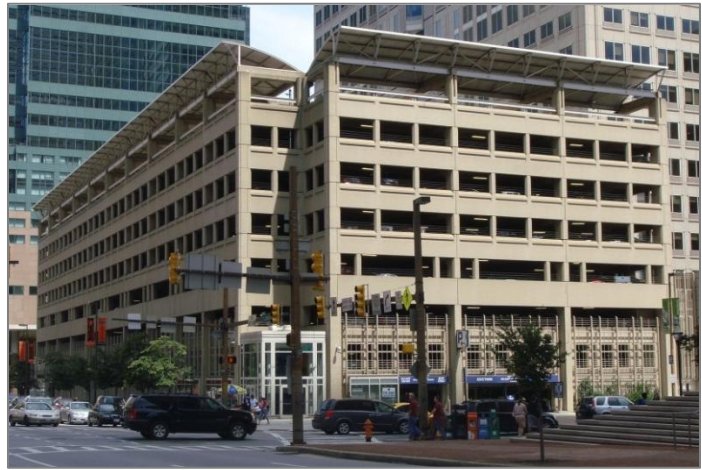
100 East Pratt Street Garage
