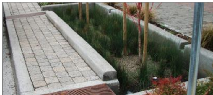
Example of a Stormwater Management Planter Cell
