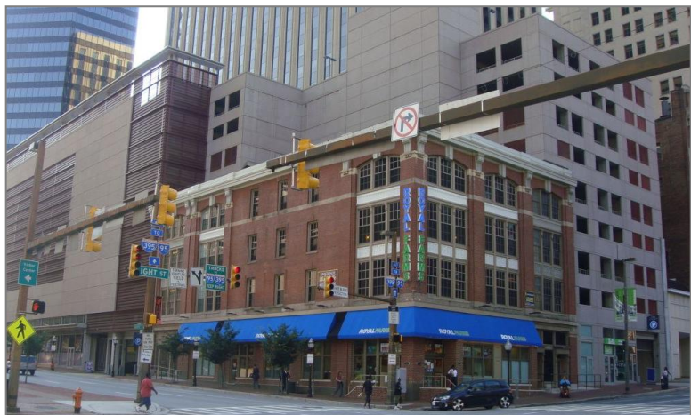
30 Light Street Parking Garage (flanking 34-36 Light Street)
