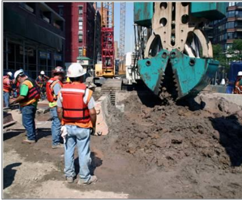
Example of activities associated with slurry wall excavation
