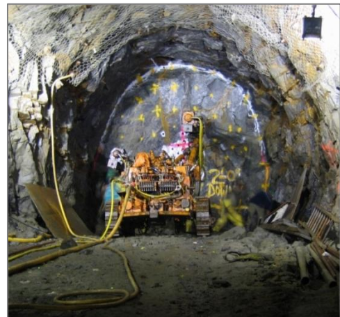
Example of drilling and blasting process
