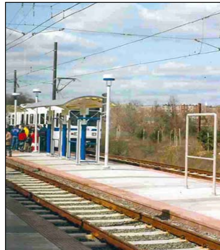
Overhead Catenary Wire System, Baltimore City
