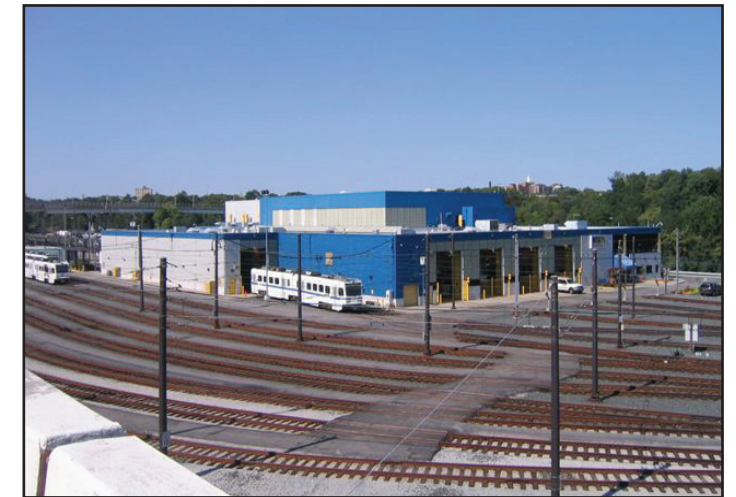
North Avenue LRT Facility
