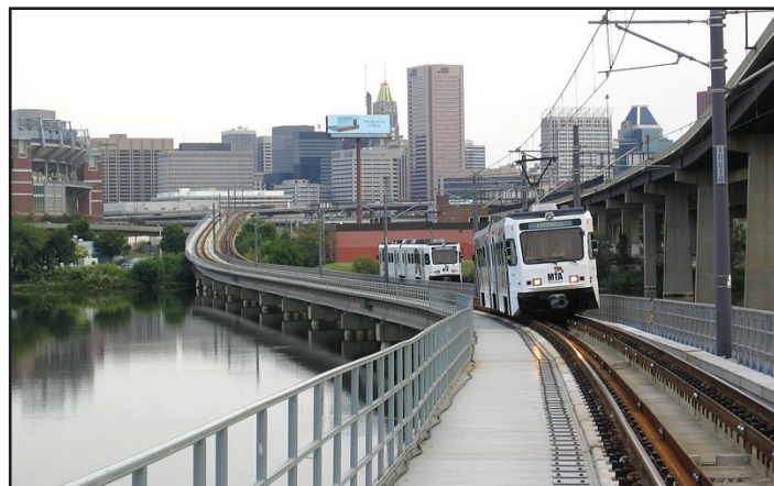
Existing Baltimore Light Rail on Aerial Structure
