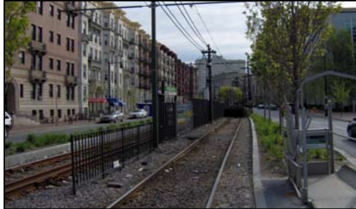
Tunnel Portal, Boston Green Line
