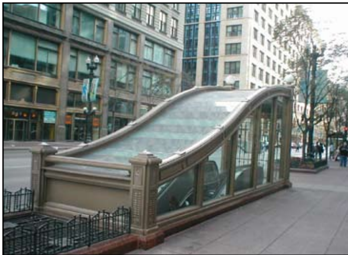
Station Headhouse, Chicago Red Line
